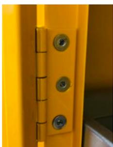
Some cabinets use rivets to attach the hinges, with just 2 hinges per door.
