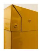
Some cabinets are riveted or spot welded and are **NOT** welded along the full length of the joint seam.
